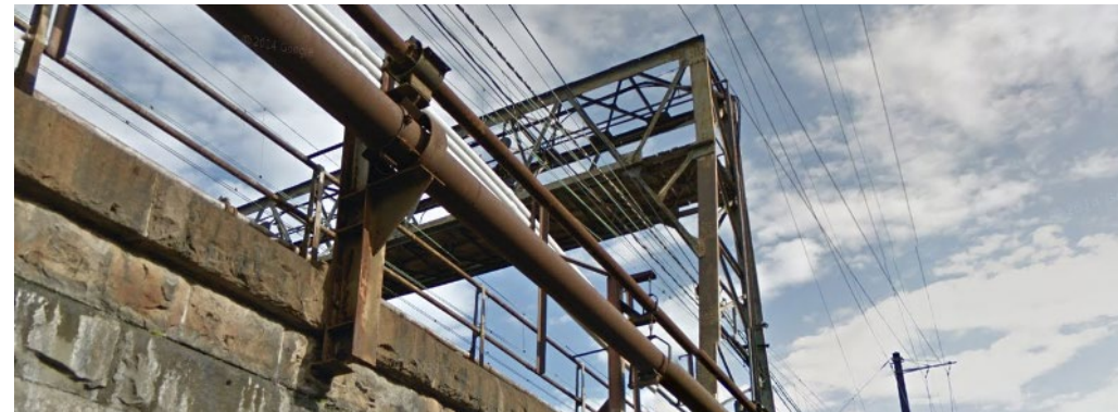
10 - CLOSE UP OF RAILROAD SIGNAL BRIDGE ON 3RD STREET
